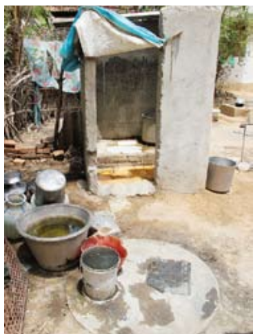
A compact soak pit toilet in Palandampatti Village.
